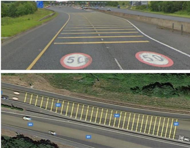
Figure 4. Example of speed limit roundels and warning yellow bars on the approach to toll plaza (source: Google Maps)
