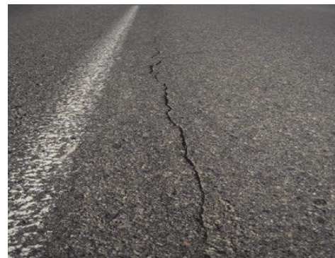
Figure 1. Longitudinal Cracking
