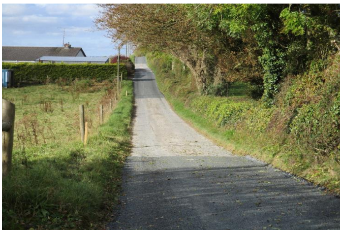
Figure 1: Visual of Site Trial during construction
