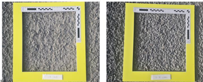
Figure 5: Visual Comparison of section constructed using reference bitumen emulsion (left) and emulsion containing the CDML additive (right) at a rate of spread of 1.7 \text{ l/m}^2
