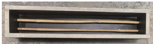
Figure 10. Formwork and bamboo culms for the concrete beams in Phase IV.
