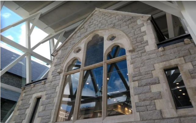
Figure 2: View of existing Church Hall structure enclosed within the new multi-story structure – photo by author.
