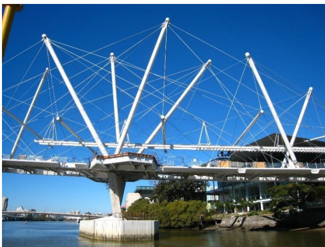
Figure 1. Kurilpa Bridge in Brisbane, Australia [2]
