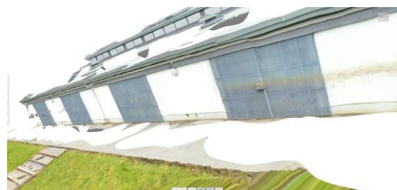
Figure 7. Photogrammetric model of the surveyed building.
