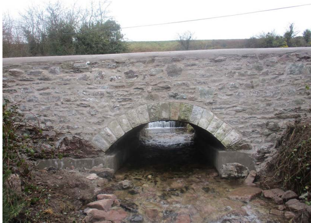
Figure 4. Ballybrogan Bridge after completion of rehabilitation works
