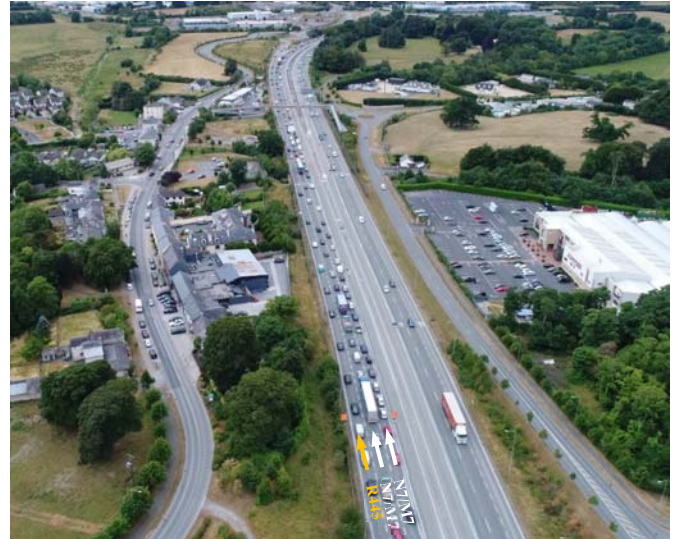
Figure 2. View of lane drop from UAV: Lane 1 (R445) exits to Naas (centre background), Lanes 2&3 (N7/M7) continue to southwest
