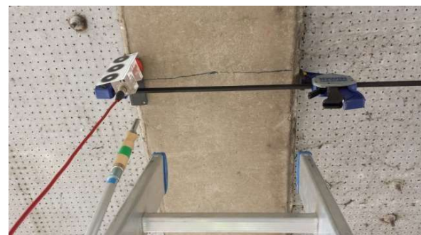
Figure 5. Instrumentation on the underside of the bridge beam.
