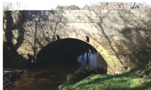
Figure 2: Segmental circular arch Bridge No. 2
